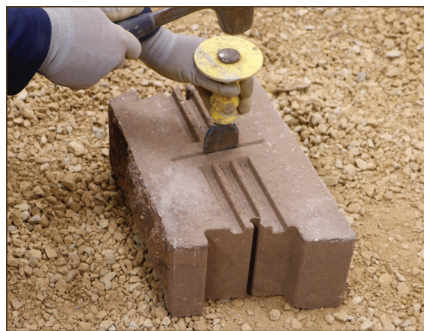
Diagram 17—Split block in half
