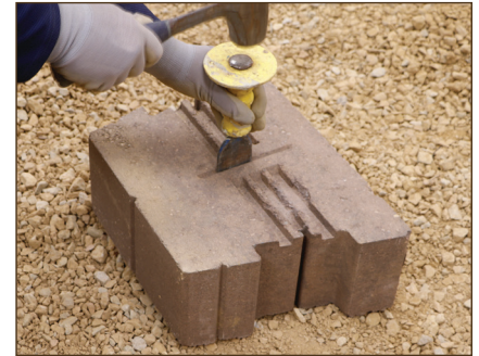
Diagram 10—Split a full size block in half
