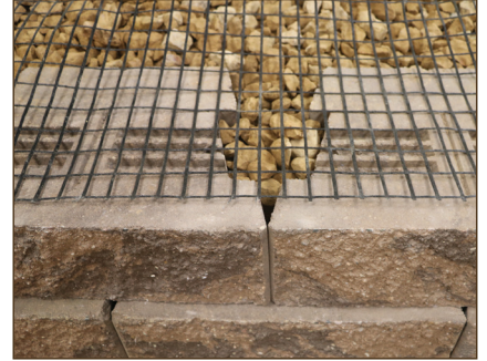
Diagram 9—Reinforcement
