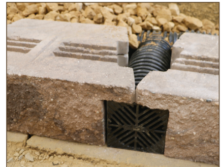
Diagram 7—Drain Pipe Placement
