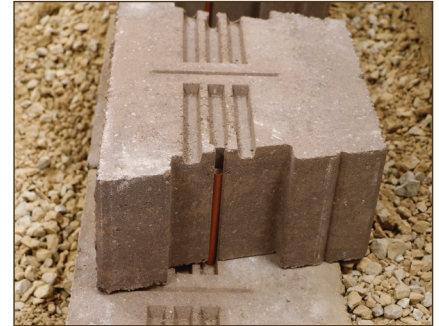
Diagram 5—Pin Placement (Battered Channel)
