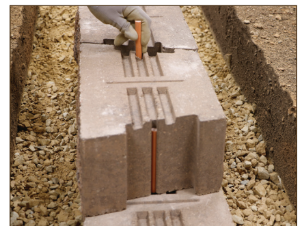
Diagram 16—Pin Placement
