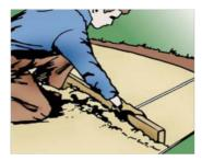
The top of the pipes should be 1 3/4" to 2" below the line. If necessary, adjust the height by putting a handful of sand under each end of the pipe if too low or by trimming the base if too high.
