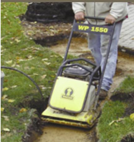
*Suitable for compaction of mixed-granular soils in a very small area.*
