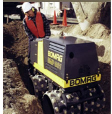
*Designed for the compaction of a wide range of soil types. This multipurpose compactor can be used for tasks like base preparation.*
