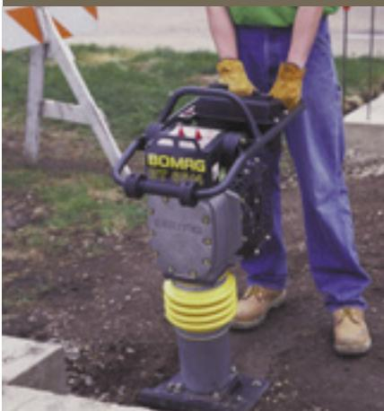
*Designed for the compaction of granular and mixed soils. Their light-weight and compact design allows these machines to work in confined areas. They can only compact very small lifts of soil (3 to 4 inches).*
